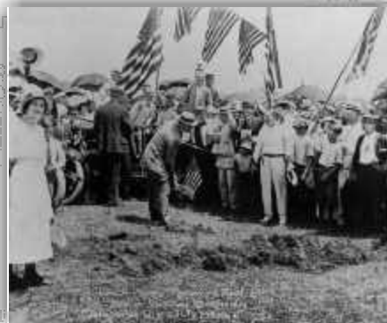
Governor Lee Cruce breaking ground for the State Capitol, Oklahoma City, July 20, 1914
